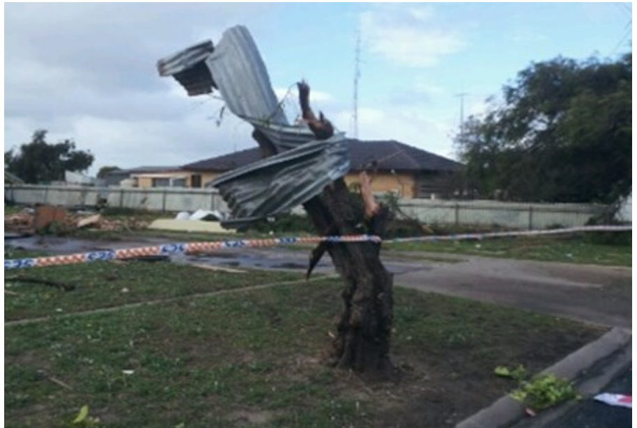
A piece of a roof wrapped around what is left of a tree
